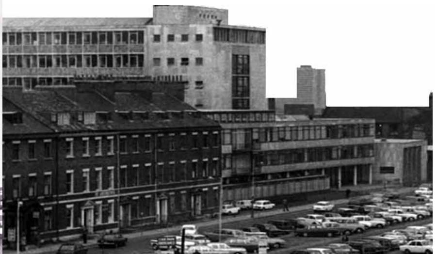
New physics building at Newcastle University in 1960s &, right the then Newcastle Polytechnic on Ellison Place. The expansion of both campuses destroyed much housing.
